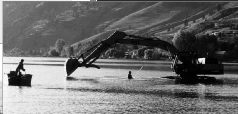
Trenching in Okanagan Lake.
