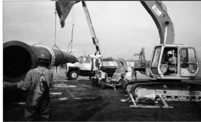
Fusing 30" pipe in Nanaimo
