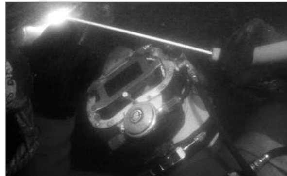
Welding an anode on a barge
