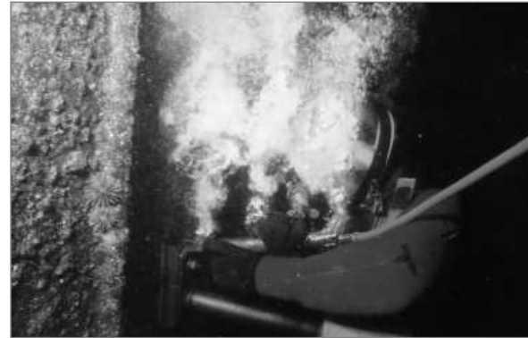
Preparing to weld a 300 pound anode on an H pile.
