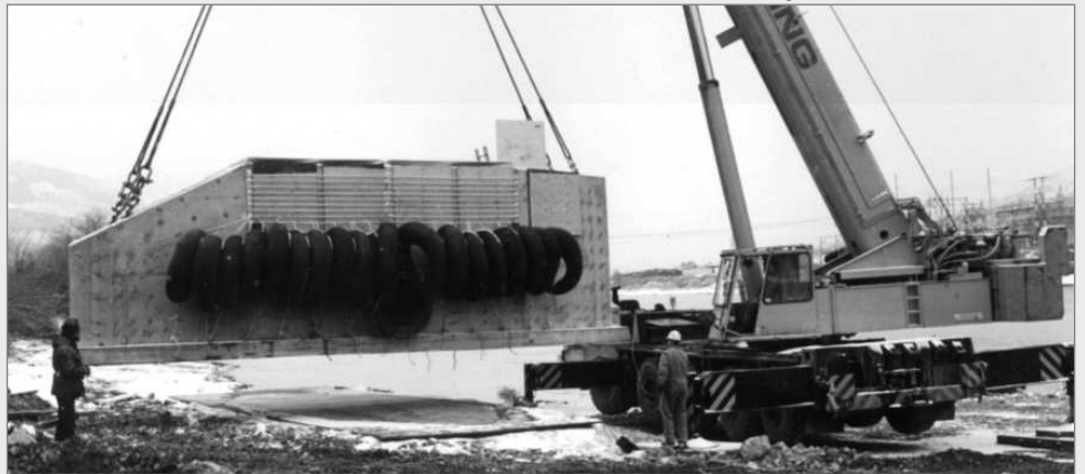
Placing 70 ton concrete intake structure.
