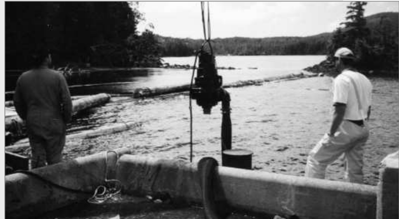
Lowering the pump to the sea bed
